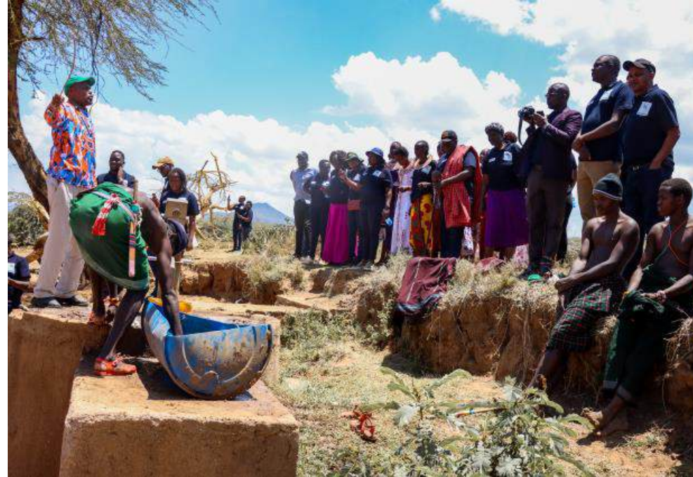
Sand dams constructed by the community
